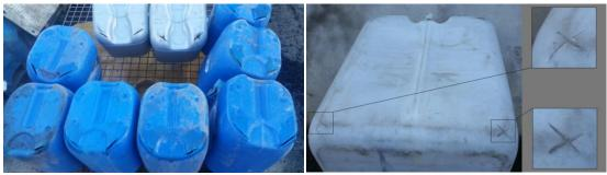
Step 2. Place upright on a slopping mesh/grate over a holding tank or similar. Then allow enough time to fully drain away, particularly oil containers, we recommend draining overnight.
